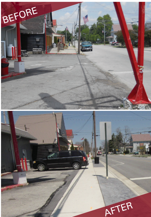
Village of Waynesfield Street Replacement
